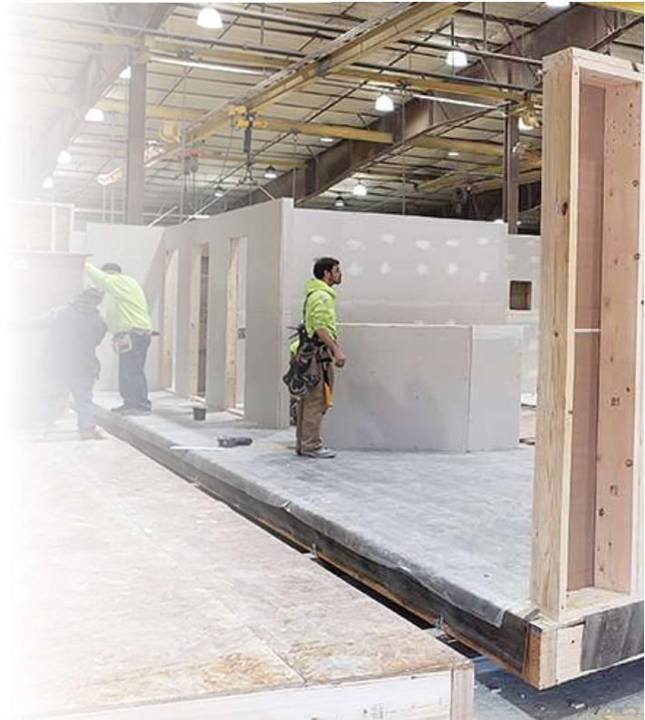
Increasingly manufacturing techniques are becoming commonplace within construction. Prefabrication and offsite manufacturing seeks to create construction components and assemblies in a controlled environment offsite before components transported to final destination for installation onsite. The aim is to reduce material, overhead, and labour costs relative to traditional construction techniques.
