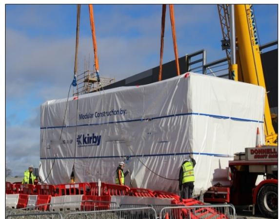
3D design and component standardisation were critical to the project's success. The modules were designed to be built in an off-site manufacturing facility. The off-site works included the fabrication of steel frame and fitting of the structural floor, installation of electrical equipment, such as UPSs, LV switchgear, battery racks, LV busbar installation to the perimeter of the modules, containment for LV submains, lighting, fire alarm and general services.
